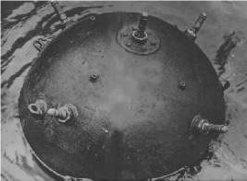
Contact mine, swept to the surface. Hit a prong and off it goes.
